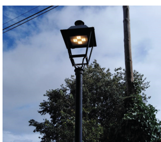
Amber retrofit installed
